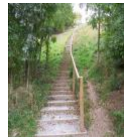
After - View of existing wooded ravine with new steps and handrails
